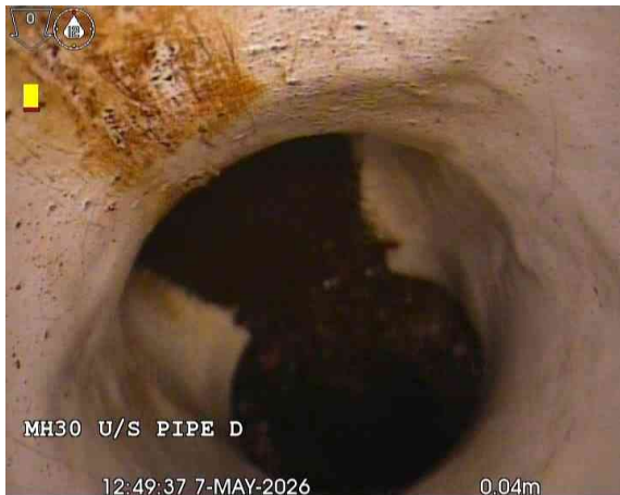
1, 00:00:10, 0.35 m Junction at 6 o'clock, 100mm dia, Buchan (winser) trap
