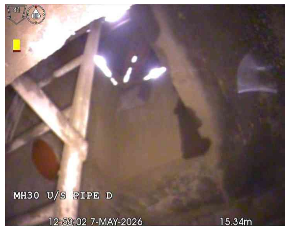
8, 00:03:32, 15.34 m Finish node, manhole, reference: SO13338904
